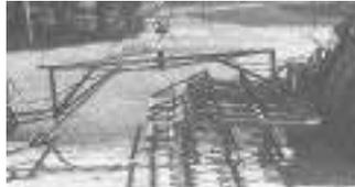
and trussed with 3/4-in. dia. sucker rod on top and bottom.
