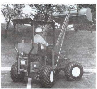
Your readers may be interested in this new "Hydra-Quad" tractor that I built. This 4-WD. 4-wheel-steer tractor is powered by a 24 hp rear-mounted gas engine and steered with a pedal foot control. Its design permits an incredibly tight inside turning circle of only 68 in. and it's equipped with 12 by 12 by 26 flotation tires which help make it an all terrain utility tractor. It has a solid front axle and an oscillating rear axle with 4 in, deflection. The
