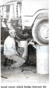
metal ramps which bridge between the wall and the pedestals are adjustable to the different widths between wheels of each individual vehicle. They are also removable for ease in working under vehicles.
