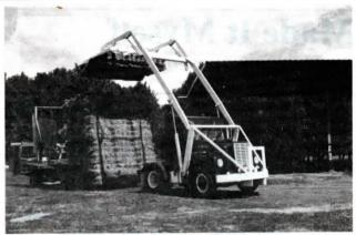
power the boom. He added ballast to the front bumper to balance the load and also installed a 10-ft. wide hydraulic-controlled angle snowplow in front.
