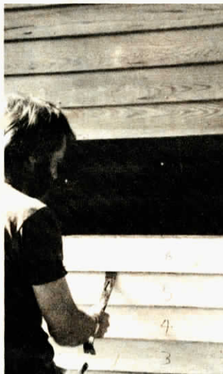
Each strip of siding was numbered so Maxwell could put it back in the same place.
