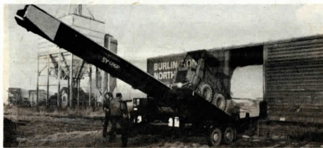
Skid-steer loader rides above hopper and, as grain empties out, it drives across tire ramps and into the box car.
