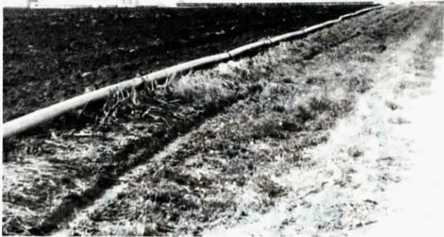
A 100-hp. high pressure manure pump moves manure through 6-in. aluminum irrigation pipe to fields up to 1½ miles away.
