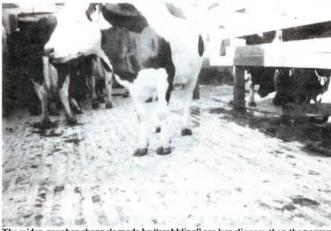
The wider, rougher channels made by "scabbling" are less slippery than the narrow grooves made by saws, says Floyd Graber.
