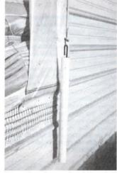
We use these homemade weights to hold down the curtain closing cables on our turkey barns. We made 16 of them in all. They're made of 24-in. lengths of 1 1/2-in. dia. pvc filled with concrete and with a bent piece of 1/4-in. rod inserted in one end as a hook. The weights are attractive yet they don't scratch up the sides of the building. (Melvin Miller, Rt. 1, Ewing, Ill. 62836)
