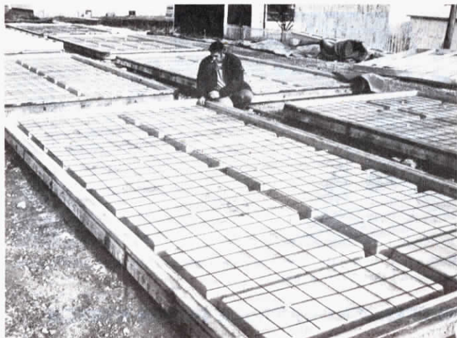
Waffle-Crete panels are 50% lighter than conventional 8-in. concrete walls.
