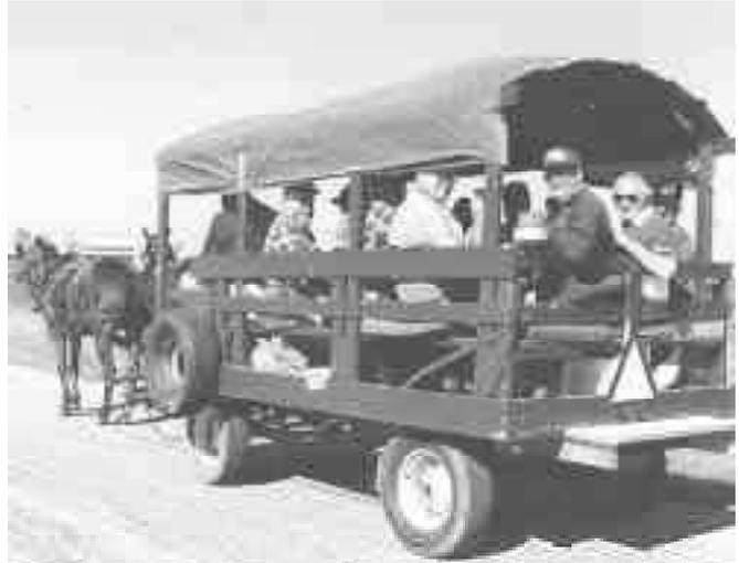
The wagon is equipped with the running gear out of a 1938 Ford car and fitted with 15-in. wheels.
