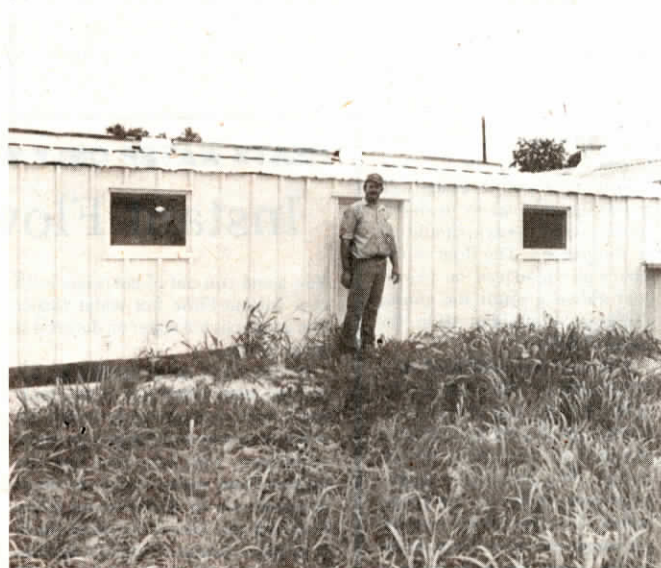
Gary Holt built nursery from 3 trailers placed side by side. Each trailer holds 90 pigs.
