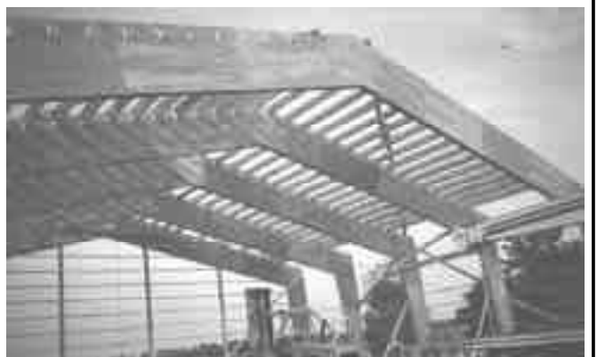
Eagle's wood frame buildings with no trusses boast many advantages over steel frame buildings, including leaving no place for pest birds to land on.
