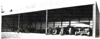
Shed is 16 ft. high in front and 13 ft. high at rear. Heinze welded 3 by 3-in. 10 ga. steel rafter plates, spaced 2 ft. apart, onto each rafter and drilled holes into them before lifting them into place with a crane. The 2 by 4 purlins are bolted to the plates.
