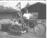
Makes it a lot of fun to ride together, and you can see him which is much safer than having him behind you. A shoulder hamess and crossbar keeps the child safe and he has a canopy over him for shade. The unit mounts on a 20-in. pneumatic tire for a soft ride. It snaps on or off the bike by removing a pair of pins from a bracket that fastens permanently to the bike. If you tip over, the Tiny Toter stays upright because of a pivot design built into the hitch.
