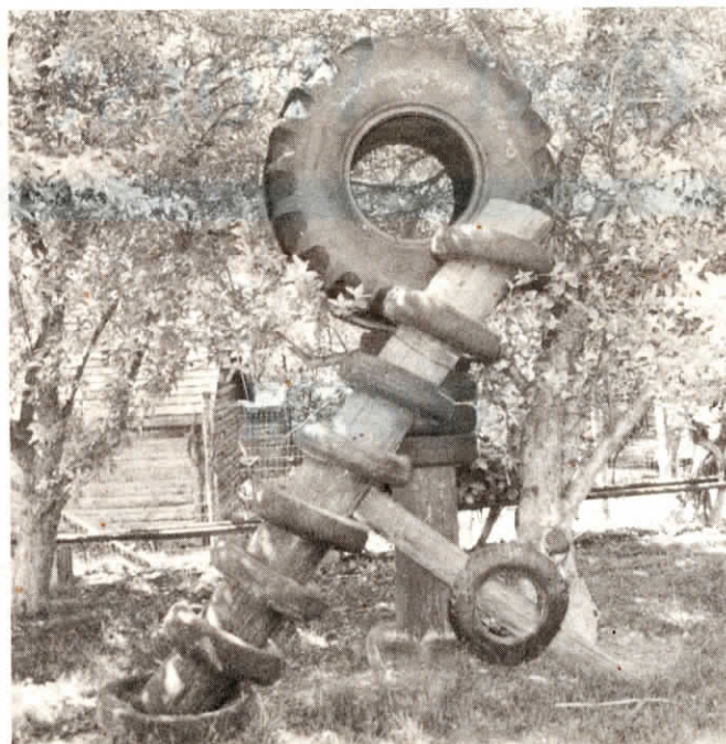
Steps made from car tires lead up to tire playhouse bolted to top of post.
