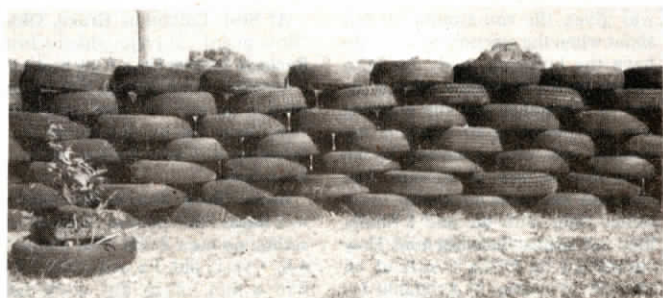
Tires aren't secured by anything other than their own weight.
