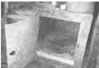
by 8 lumber and 3/4 in. plywood. The mailbox is protected inside the wood, just under the top 2 by 8. For the post, we used a railroad tie and fitted it with heavy-duty door hinges. The protector swings one way, and a heavy spring brings it back. A plastic newspaper delivery box bolts to the outside of the housing. (Richard Marley, 445 County Rd. 2500 N., Mahomet, Ill. 61853 ph 217 359-8570)
