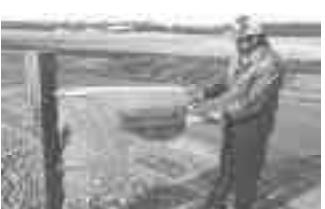
After a lot of trouble with vandals and snowplows, we finally decided to build this heavy-duty hinged mailbox protector. First we made a triangular-shaped housing out of 2
