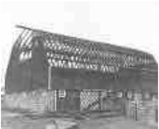
After removal of barn roof (left), local carpenters easily install new clear span roof.
