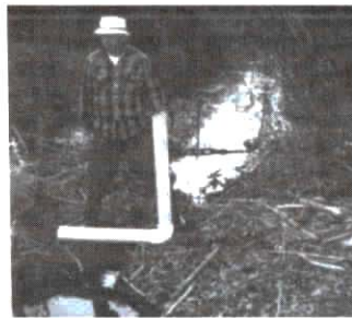
L-shaped PVC pipe is part of the "final solution" for pesky beavers.
