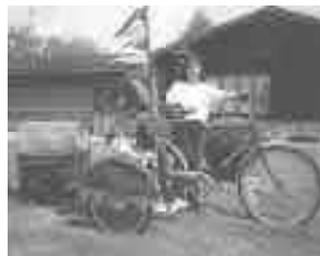
Makes it a lot of fun to ride together, and you can see him which is much safer than having him behind you. A shoulder harness and crossbar keeps the child safe and he has a canopy over him for shade. The unit mounts on a 20-in. pneumatic tire for a soft ride. It snaps on or off the bike by removing a pair of pins from a bracket that fastens permanently to the bike. If you tip over, the Tiny Toter stays upright because of a pivot design built into the hitch.
