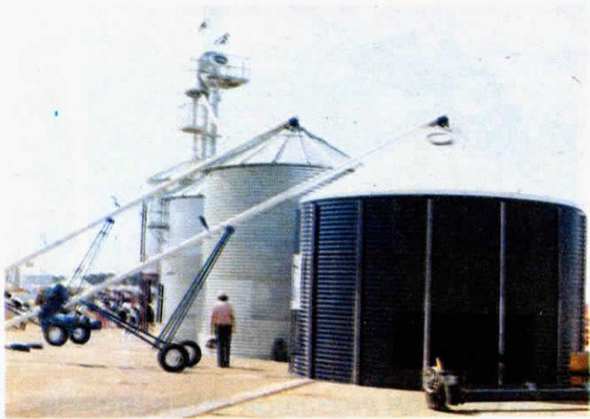
Bin walls are made of corrugated steel (4 in. wide corrugations) and lined on the inside with glass fused to steel.
