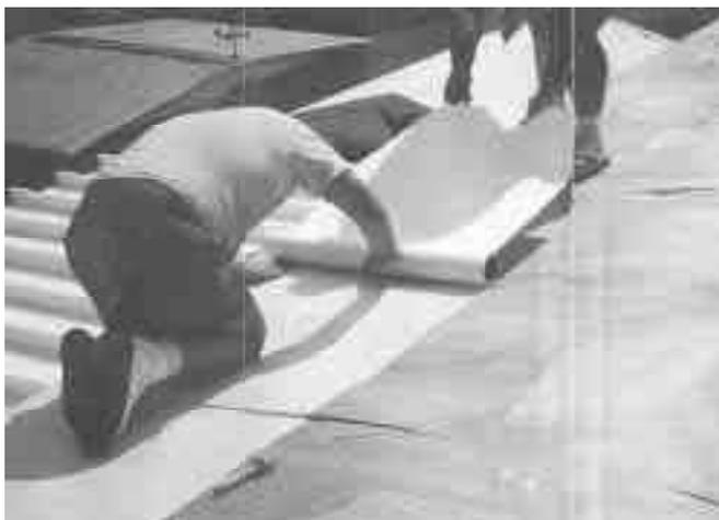
You apply the self-adhering, aluminum-faced roll roof material by peeling off the paper backing and sticking it down to any clean, dry surface, including old asphalt.
