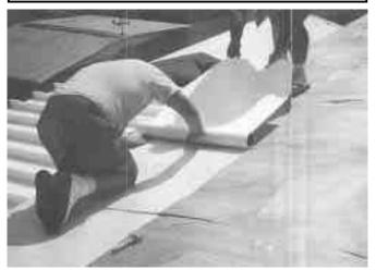
You apply the self-adhering, aluminum-faced roll roof material by peeling off the paper backing and sticking it down to any clean, dry surface, including old asphalt.
