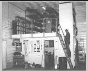
Roger & Bruce Elliott, Montrose, Ill.: "We put on a 40 by 60-ft. addition with 16-ft. of clearance in 1992 so we could pull combines inside to work on them," explains Roger. "The extra ceiling height also allowed us to set up a handy storage area above our 10 by 12-ft. office, which we built in one corner of the addition."
