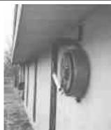
Bracket that holds tube swings out of the way and extends only 8 in. from wall.
