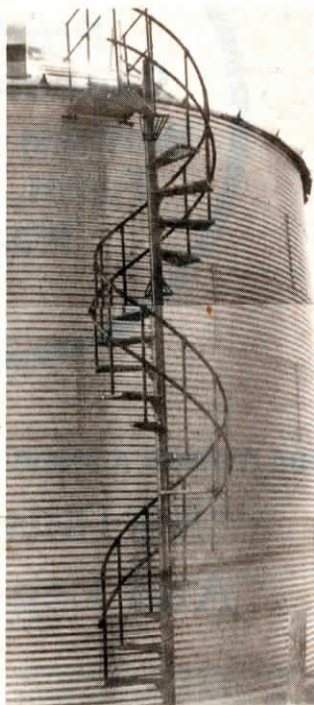
No on-site welding is required to assemble the bolt-together stairway.
