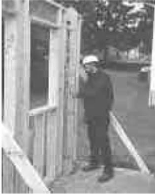
the holder by ripping a 7-in. wide sheet of 3/4-in. plywood. Then he cut out a section along one side that's 1/4 in. wider than his level. He made 45° cuts on either end to leave a small, flat point to rest on the floor. A hand hold near the center of the holder makes it easy to carry and hold in place. Four strips of duct tape hold the level in place.
