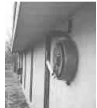
Bracket that holds tube swings out of the way and extends only 8 in. from wall.
