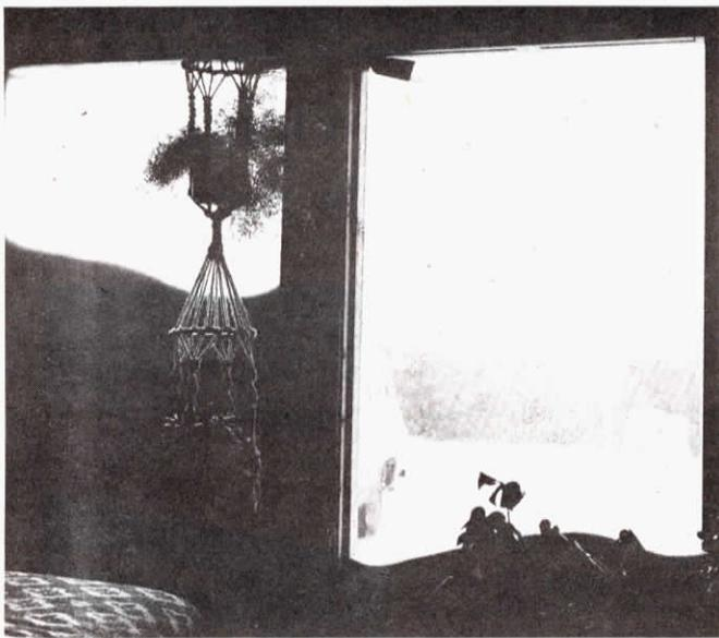
Layer of insulation beads can be blown in to fill window (as on left) or blown out to provide clear view (as on right)
