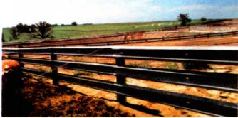
To make fencing, guard rails are lag bolted to posts spaced 12 ft. apart.
