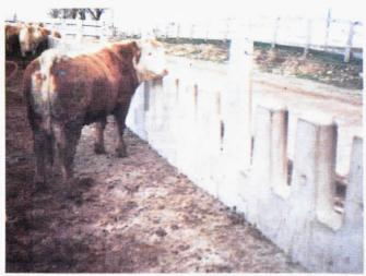
Feeder sections are 7.5 ft. long and 42 in. high. Interlocking cableholding sections are 5 ft. high, 15 in. wide.
