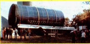
In less than six hours this 20 by 50-ft. Harvestore was down and ready to move down the road. Grotte figures that moving steel silos in one piece will cost about half as much as moving them in sections.
