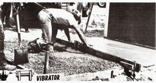
Photo shows how one man can level spans up to 20 ft. using the new Custom Vibe vibrator, shown on left. The device "walks" in the direction of the pull, allowing one man to strike the concrete by simply guiding the board
