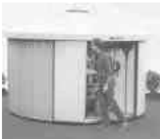
With a slight push, outside of building rotates a full 360 degrees right or left. Floor remains stationary.
