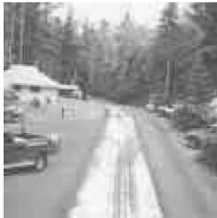
**Special acrylic polymer suppresses dust and creates a hard surface without the expense of paving or oiling.**
