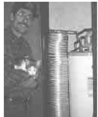
Space heater taps into hot water line and runs through stove pipe mounted on side of water heater.
