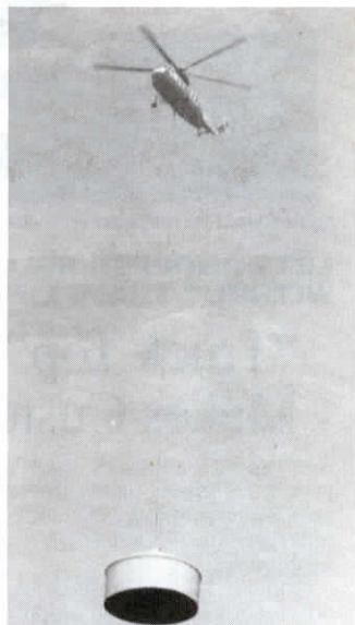
Helicopter transported each bin in sections. Bracing inside the rings kept them from collapsing inside.
