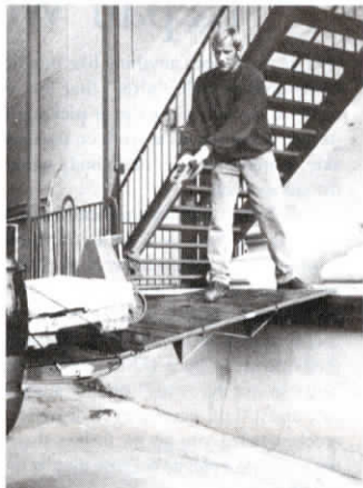
"Suspension bridge" type cable supports underside of ramp to keep it rigid.
