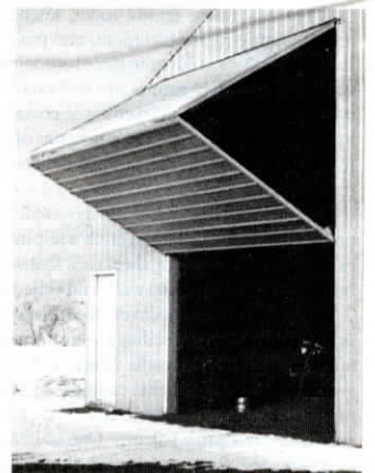
Smith's 15 ft. wide bi-fold door is powered by a variable speed electric motor that drives a worm drive gearbox that cranks up lifting cables.
