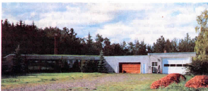
Whitehead's shop and garage attach to his home-built 2,000 sq. ft. "underground" house. Heat is provided by hot water running through 1-in. pipe imbedded in concrete floor of house.
