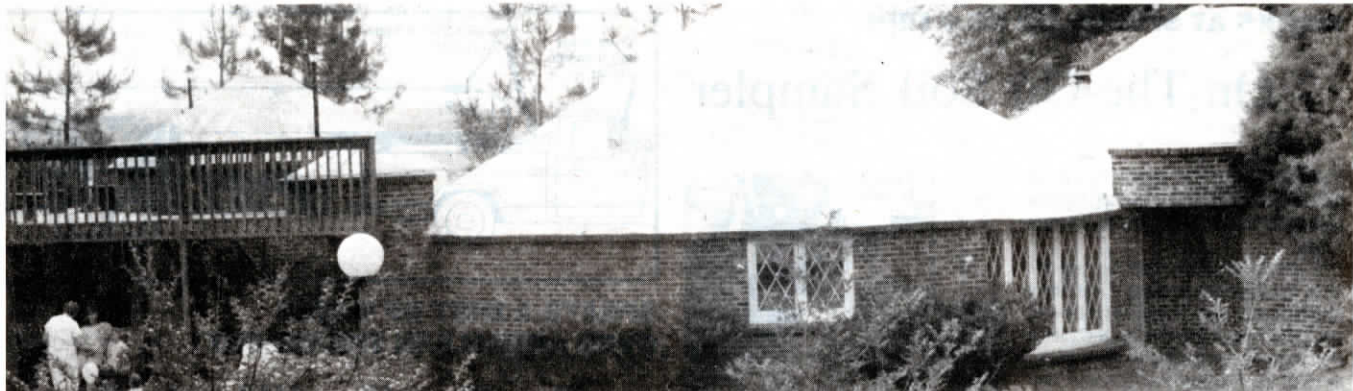
Dean Kennedy's "grain bin house" consists of two 36-ft. dia., 22-ft. high corrugated bins, placed side by side, partially buried and connected by a tunnel. Upper 8 ft. of the south sides of both bins is covered by brick. Each bin has its own entrance covered by a canopy built from the top of smaller bins. Storage bin and deck adjoins one bin.
