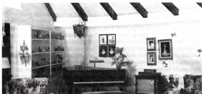
View of the family room. Interior walls are covered by sheet rock that was bent to fit the curve of the walls and nailed to 2 by 4 studs. The ceilings were formed with 6-in. sq. wood beams which arch upward toward a skylight, creating an umbrella effect.
