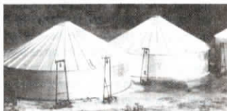
This view shows the north side of bins before they were covered by earth and cabinets.
