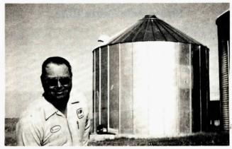
the bottom two rings, 20 ga. on the top two rings, and installed a conventional Chief roof.
