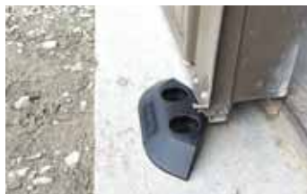
Floor guides are made from durable nylon and feature a tapered design that continually redirects doors back into proper alignment during travel.
