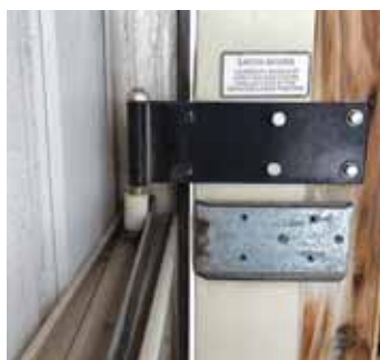
As the door reaches the final stage of travel, the roller engages the channel and gradually pulls it inward, creating a tight seal.
