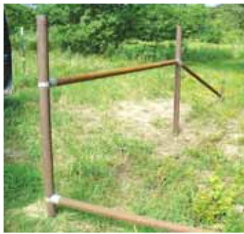
Brackets provide bracing comparable to that of a welded brace in terms of structure and integrity.
