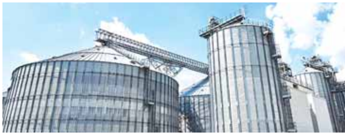
Aeration systems help operators manage airflow in large bins, while grain monitoring products track conditions that directly affect grain quality.
