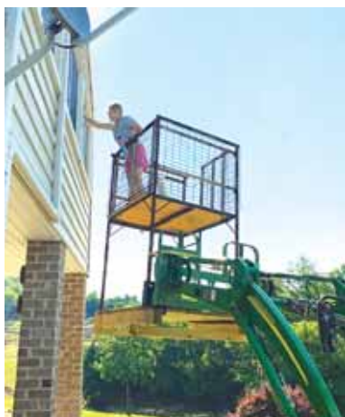
Freeman used industrial storage racking to fill in the scrap-steel frame and hangs a chain across the gate for security.
