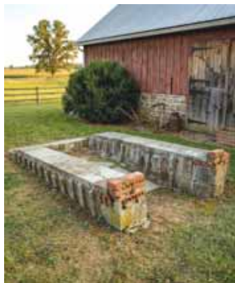
We found several versions of this outdoor service pit on a slope, built from concrete.
