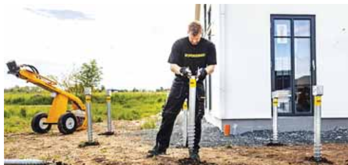
No heavy machinery, deep holes, messy concrete or long delays — just a reusable and strong foundation ready for construction right away.
