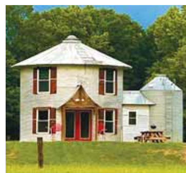
Jon Fleenor and his wife, Margaret, designed and built a two-story "bin house" from a 24-ft. dia. grain bin as part of their Katie Farms operation in Alabama.
