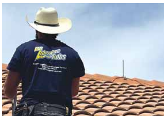
While many people believe lightning rods attract lightning, they actually provide a safe, low-resistance pathway for massive electrical charges to follow.
