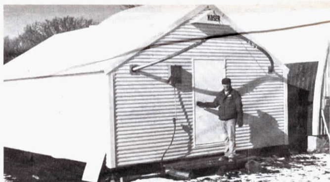
Koser's all-steel building features several industry "firsts".
