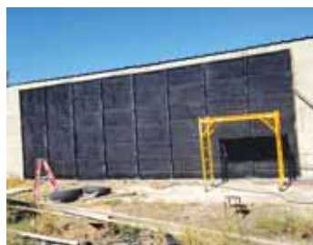
"I've got a thermostatic switch that I put at the top of the heater. When the temperature reaches 80 F, the fan cuts in and heats the shop," says Taylor.
