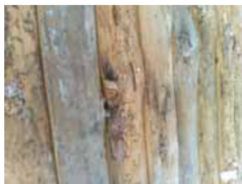
Cut pine slabs used to side sheds to protect the OSB walls.
