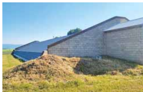
16,000-sq. ft. building was built in the 1940s or 1950s and has an 80 by 200-ft. roof with a 30-ft. high center beam. Its current metal roof was once a sod roof.
